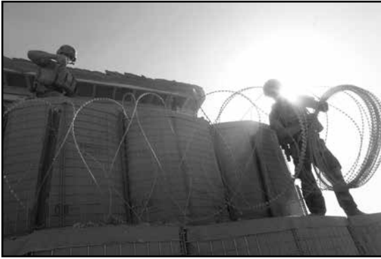
Figure 2: Engineers of U.S. Marine Corps Forces Special Operations Command (MARSOC) lay C-wire at a newly-constructed Village Stability Platform in Nahr-e Saraj district, Helmand Province. U.S. Marine Corps photo by Cpl. Kyle McNally.
